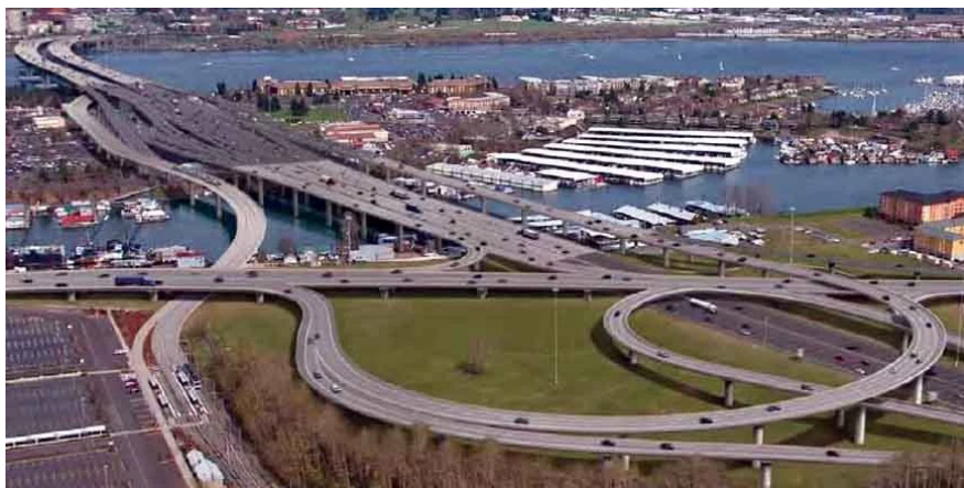
The $880 million Hayden Island/Marine Drive interchange is 17 lanes at its widest point, not counting a lane for light rail.
